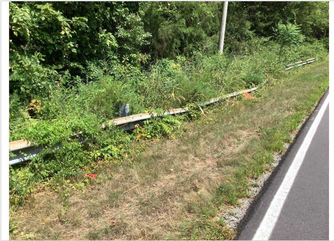
Damaged guardrail at approach #2 right
