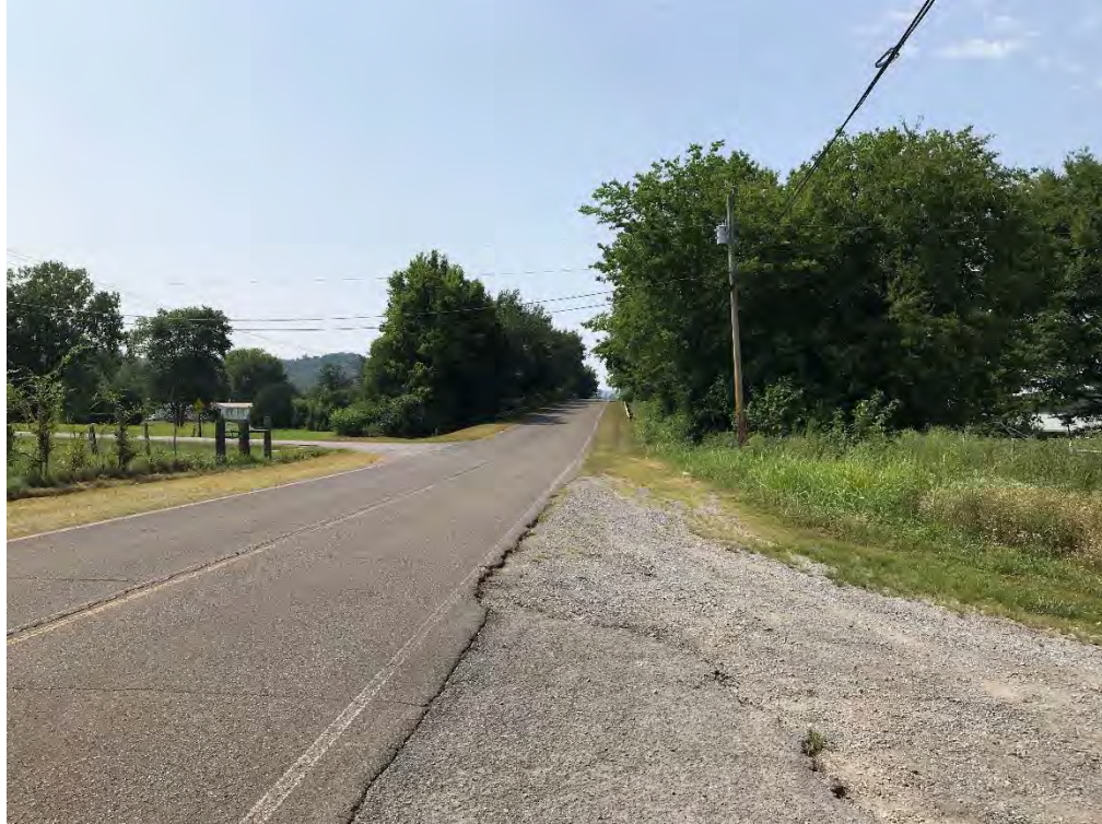
Northern Approach looking South
