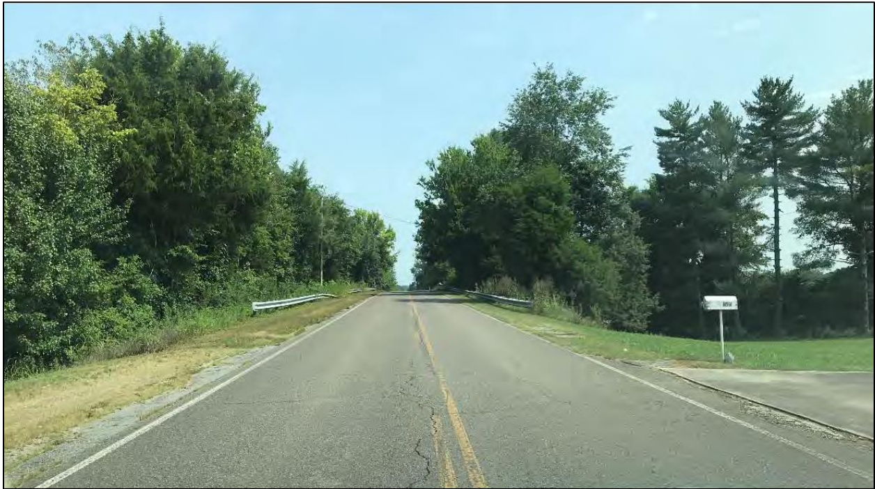
Figure 14. South approach looking north.
