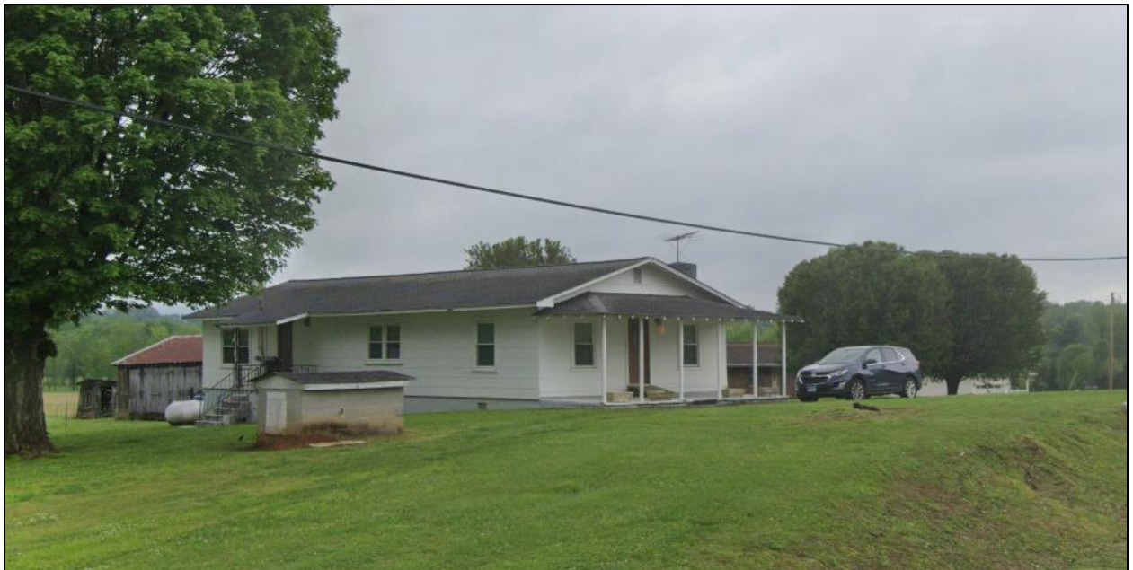
Figure 9. Southwest elevation and southeast I of MI-481, looking northwest.
