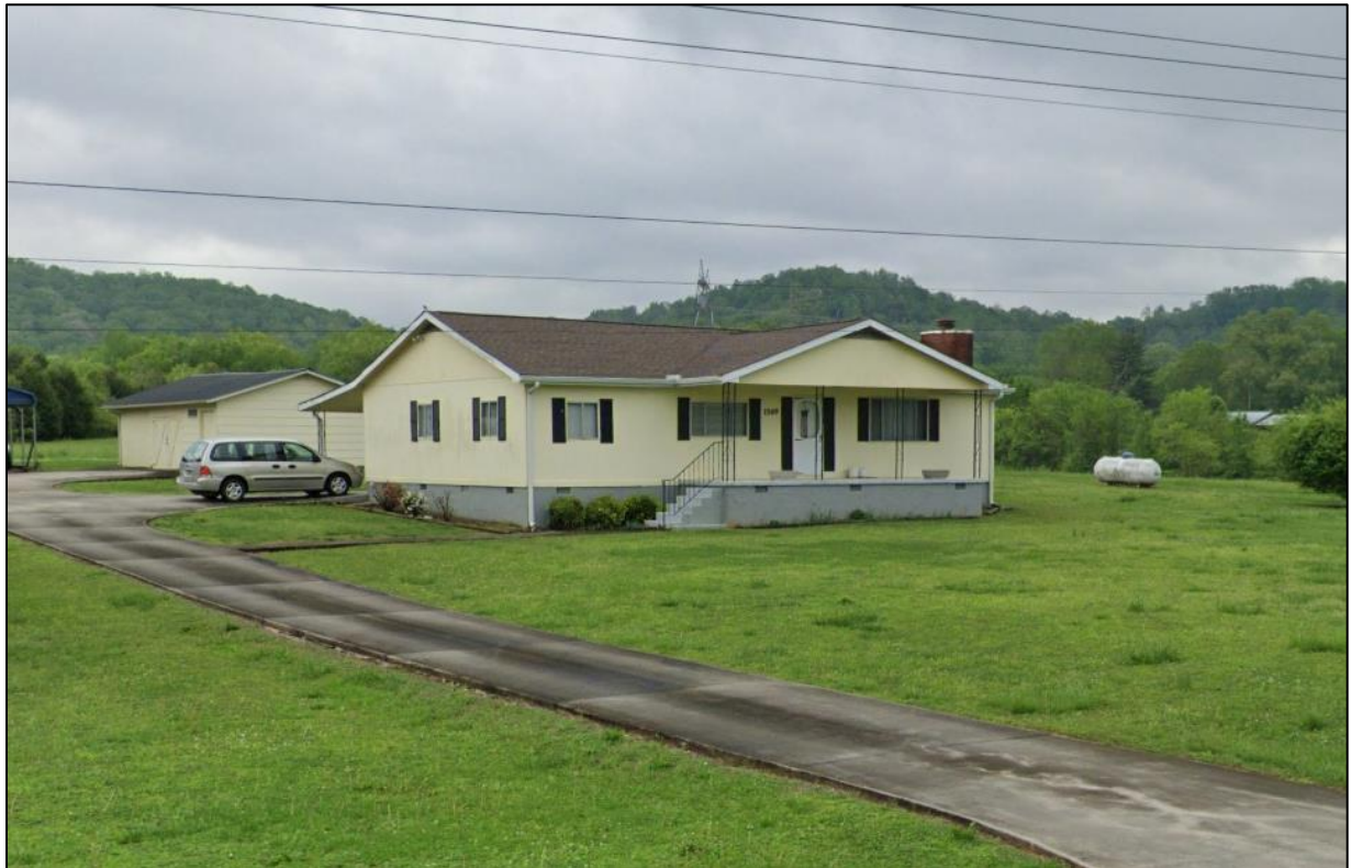
Figure 20. North elevation and west I of HS-2, looking southeast.
