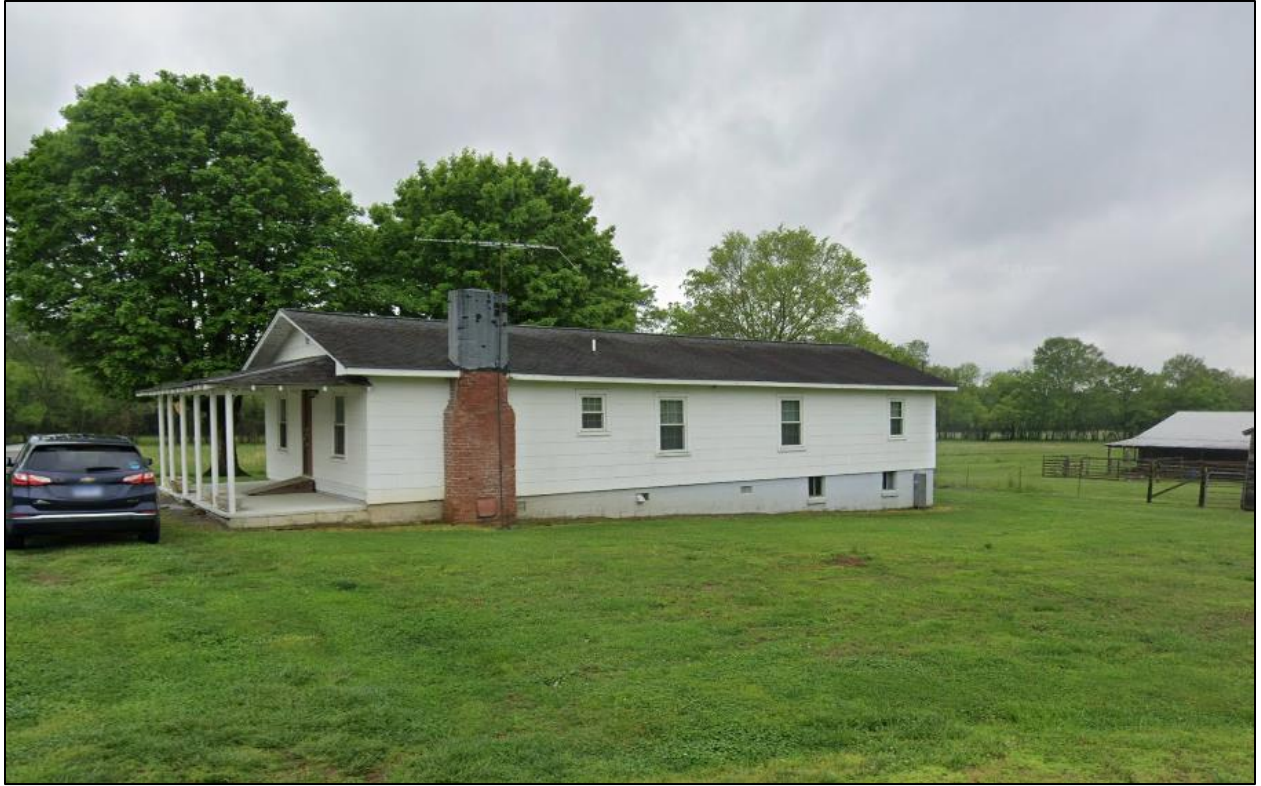
Figure 10. Northeast elevation of MI-481, looking south.
