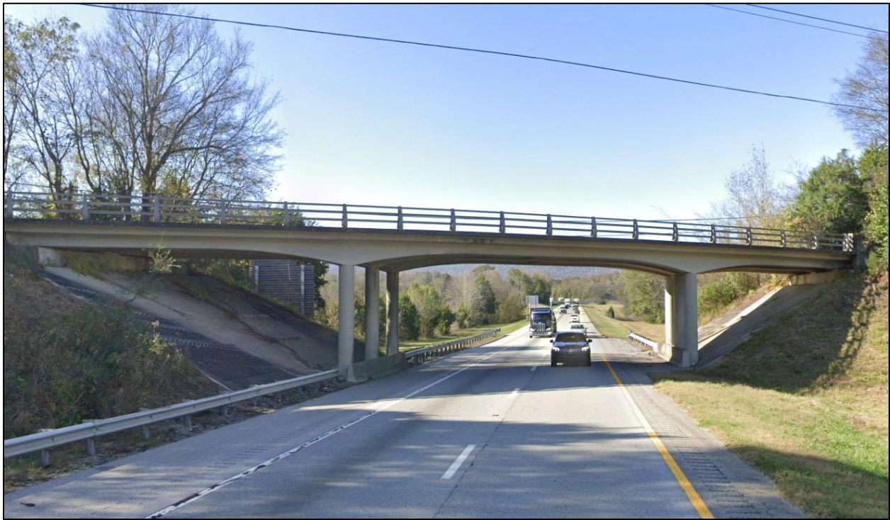
Figure 17. Looking northwest along I-24 at the current structure.
