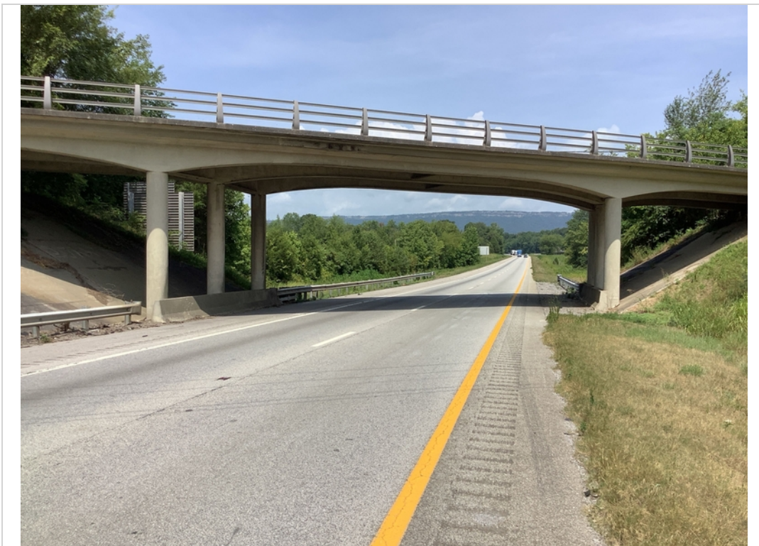
Underclearance looking back on underpass route
