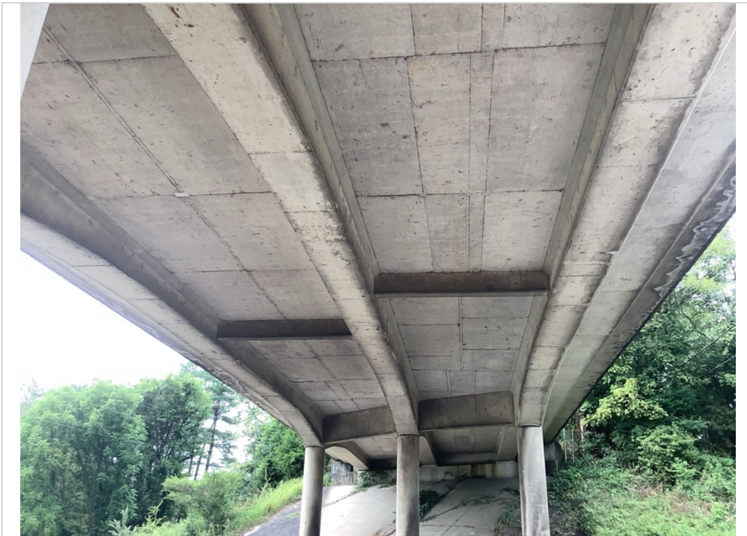
Typical bottom of deck
