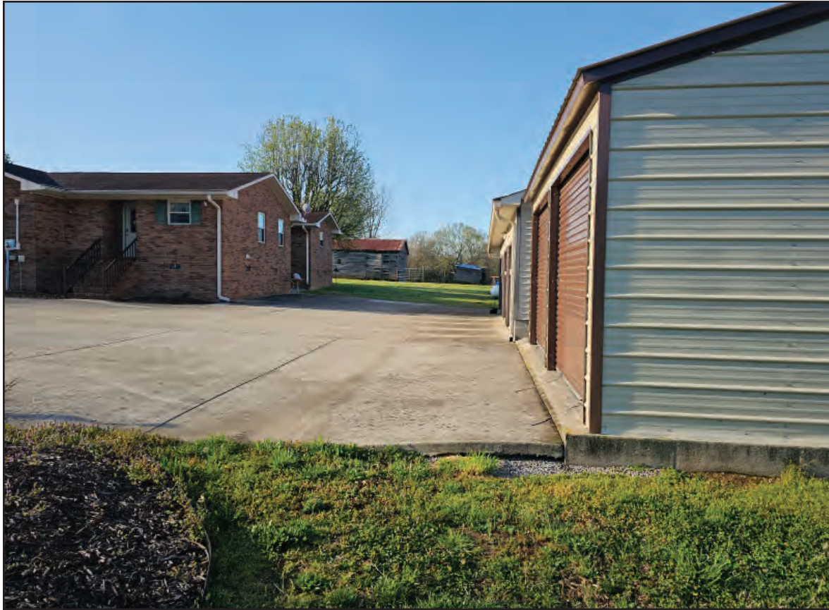
Figure 2.1. Paved driveway and building within the survey area (facing southwest).
