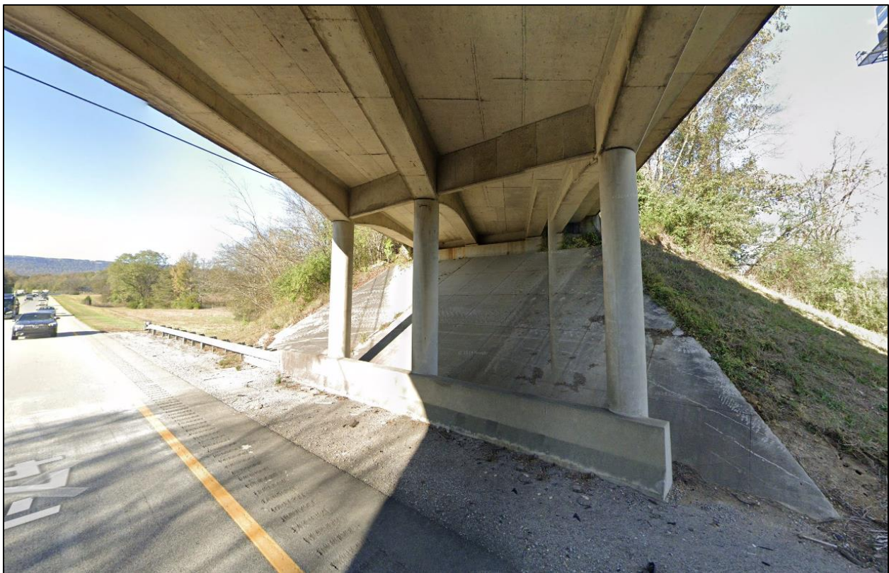
Figure 18. Looking north at the concrete girder and concrete piers.
