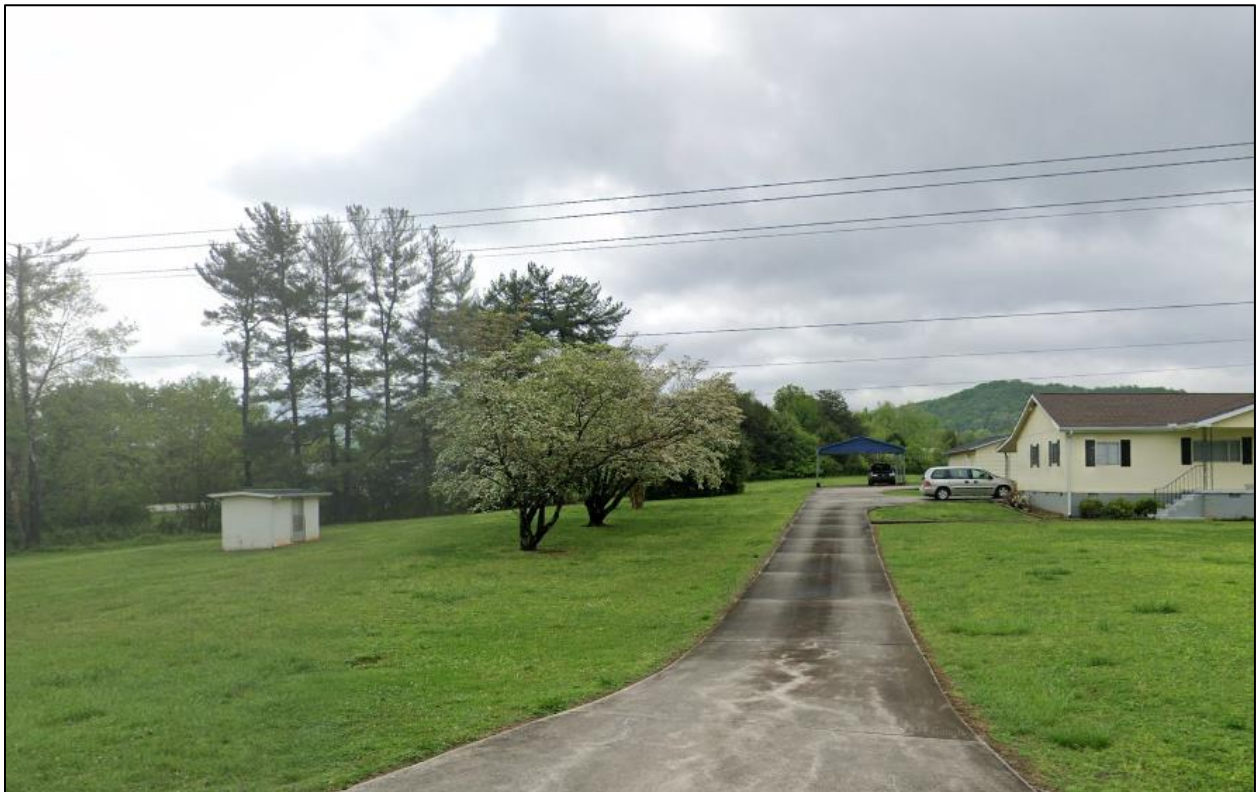
Figure 22. Concrete block outbuilding, metal carport and side-gabled garage associated with HS-2, looking northeast.
