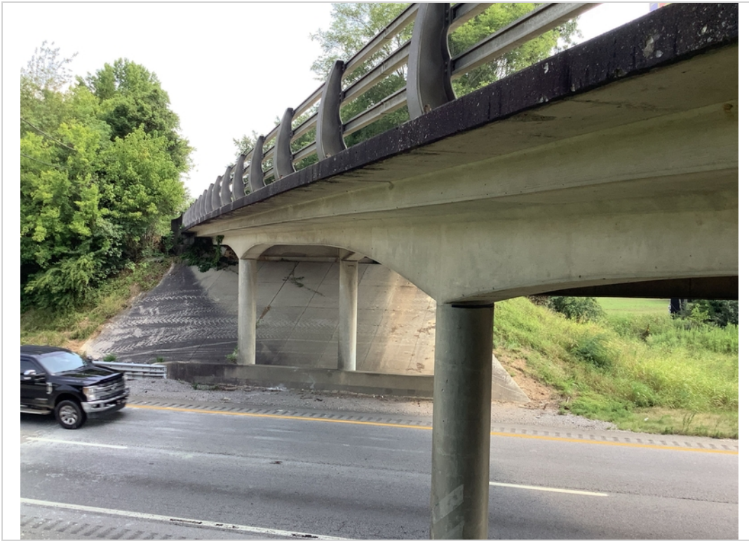
Right side view of structure
