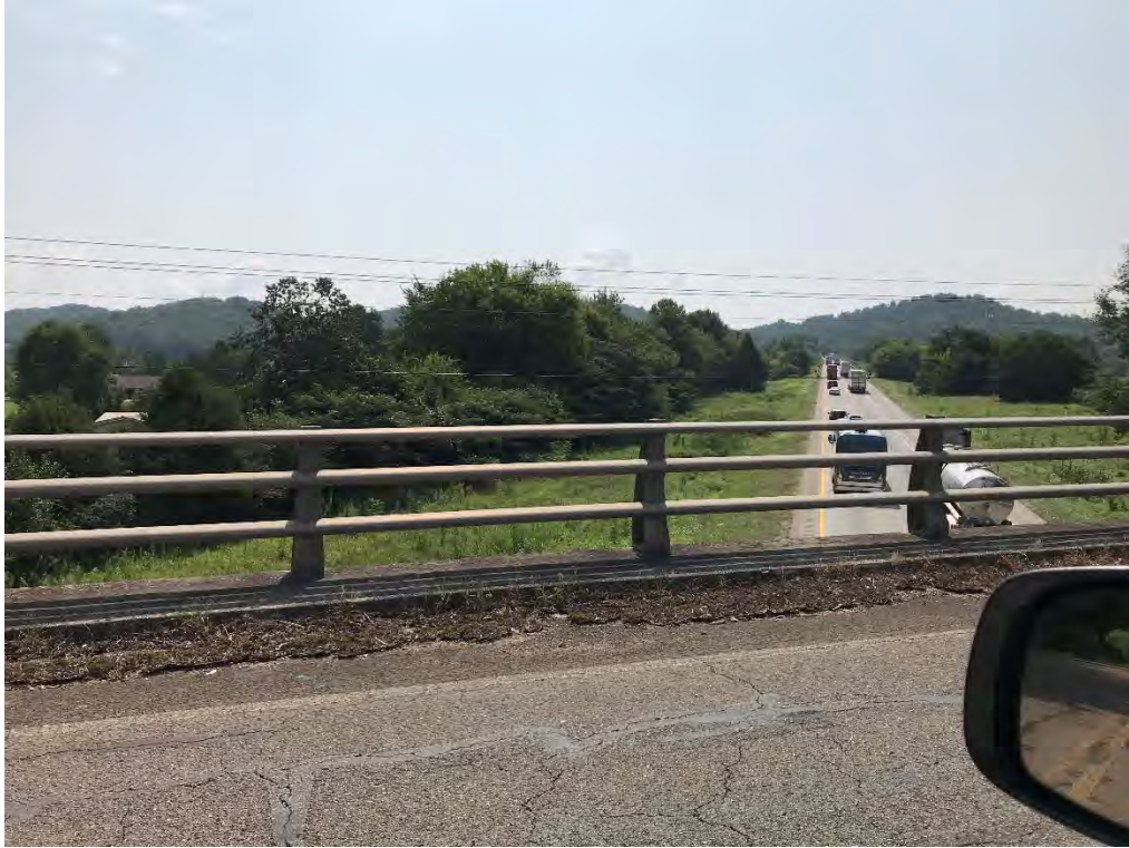
Eastern Edge of Bridge
