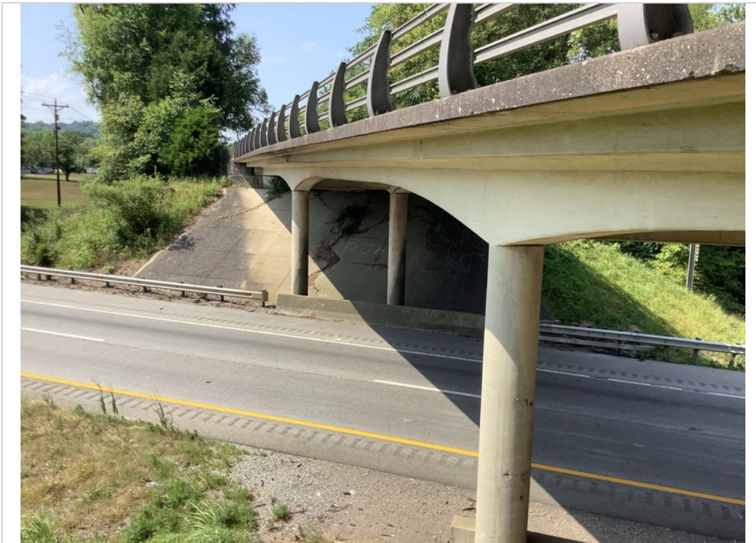
Left side view of structure
