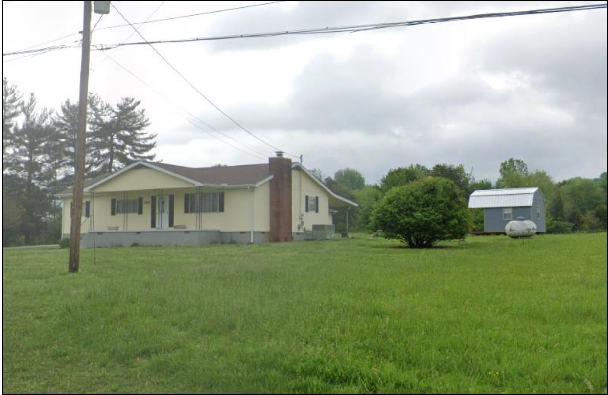
Figure 21. West and south elevation of HS-2 and associated gambrel roof shed, looking northeast.
