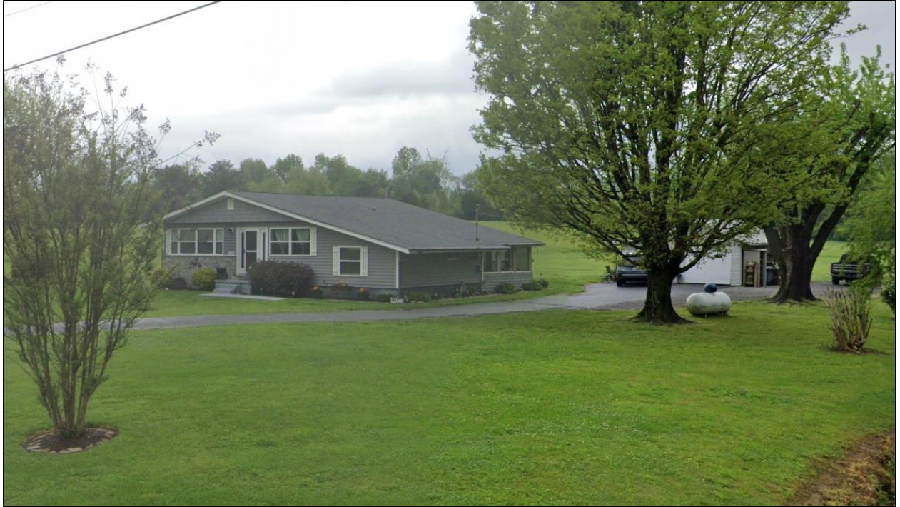
Figure 25. West I and south elevation of HS-3, looking northeast.
